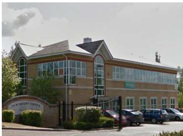
Turnhams Green offices
